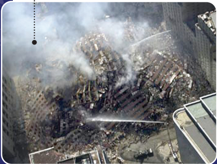
debris centered within building footprint
