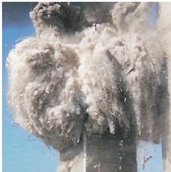
Figure 1: WTC 2 appears more like an explosion than a gravitational collapse.
